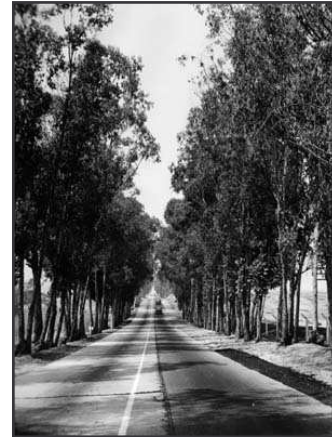
Rosecrans Avenue, looking west from Pacific Avenue, circa 1940. The Eucalyptus trees were removed in 1969 when Standard Oil Company (Chevron) agreed to widen the roadway.
