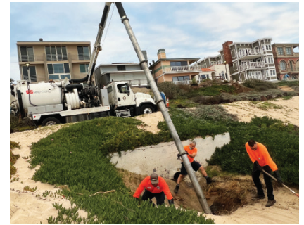
City crew vacuuming trash from storm drain outfall at beach.
