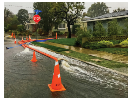
Failing storm drains cause flooding in neighborhoods, sinkholes, and private property damage.
