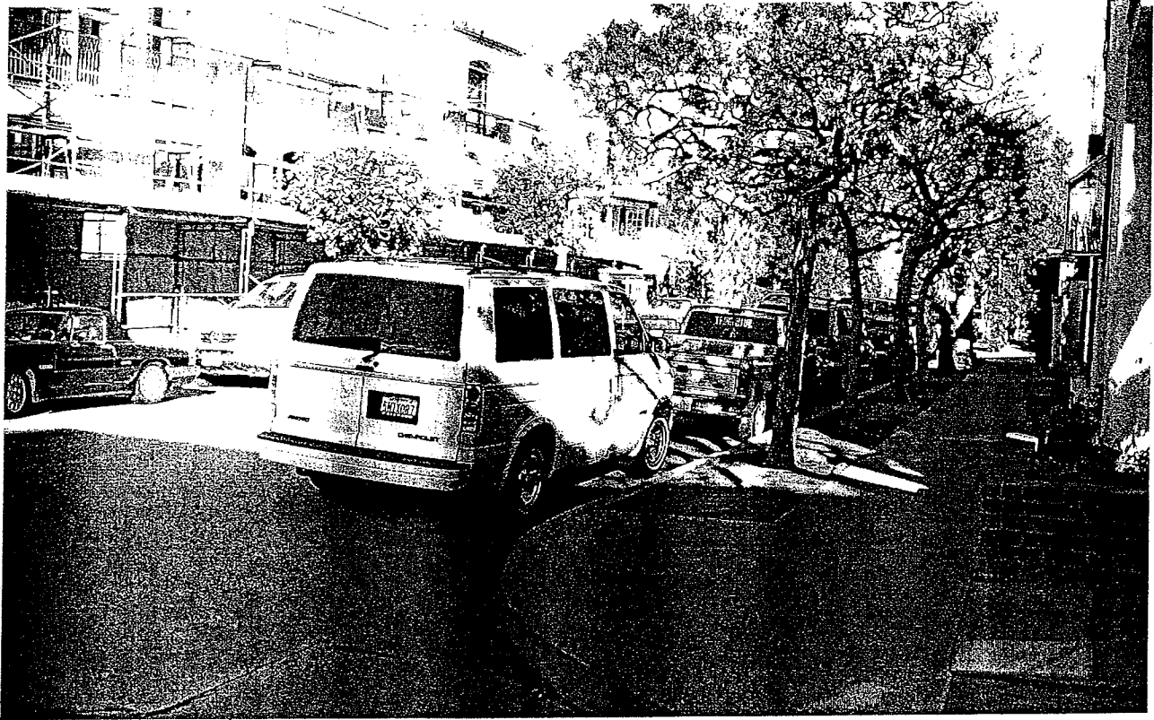
2 nd Street at Morningside Drive Looking East (South Leg)
