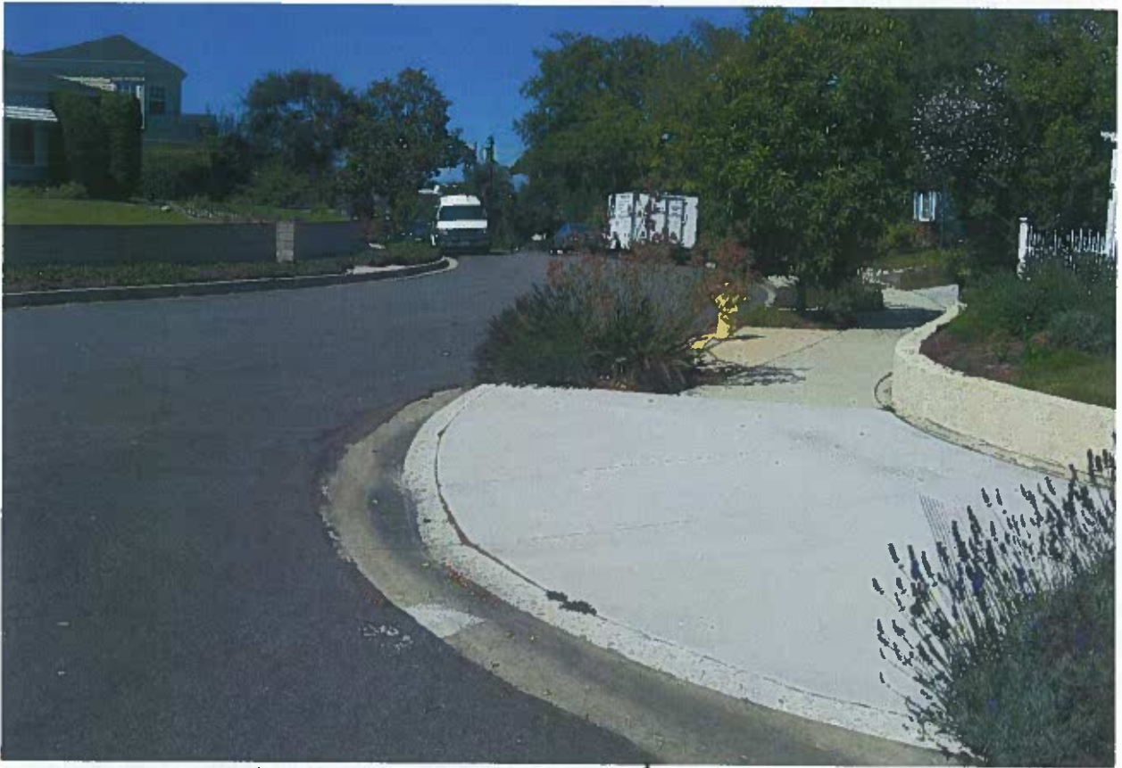
Magnolia Avenue (Southeast Leg) at 22 nd Street Looking Northeast
