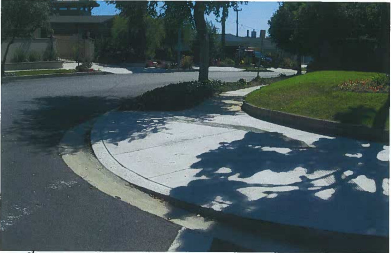
22 nd Street (Northwest Leg) at Magnolia Avenue Looking Southwest Towards 21 st Street
