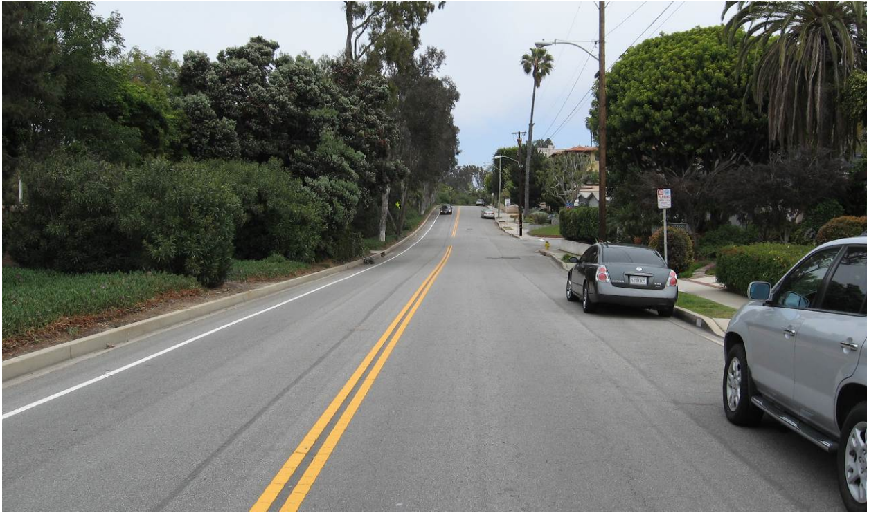
Ardmore Avenue West of Flournoy Road Looking East
