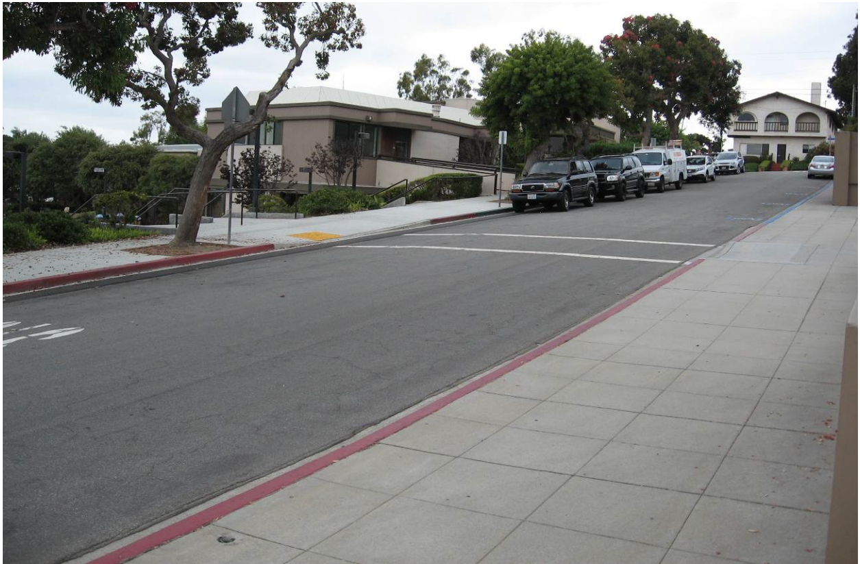
Crosswalk on Deegan Place South of 15 th Street (West Side)
