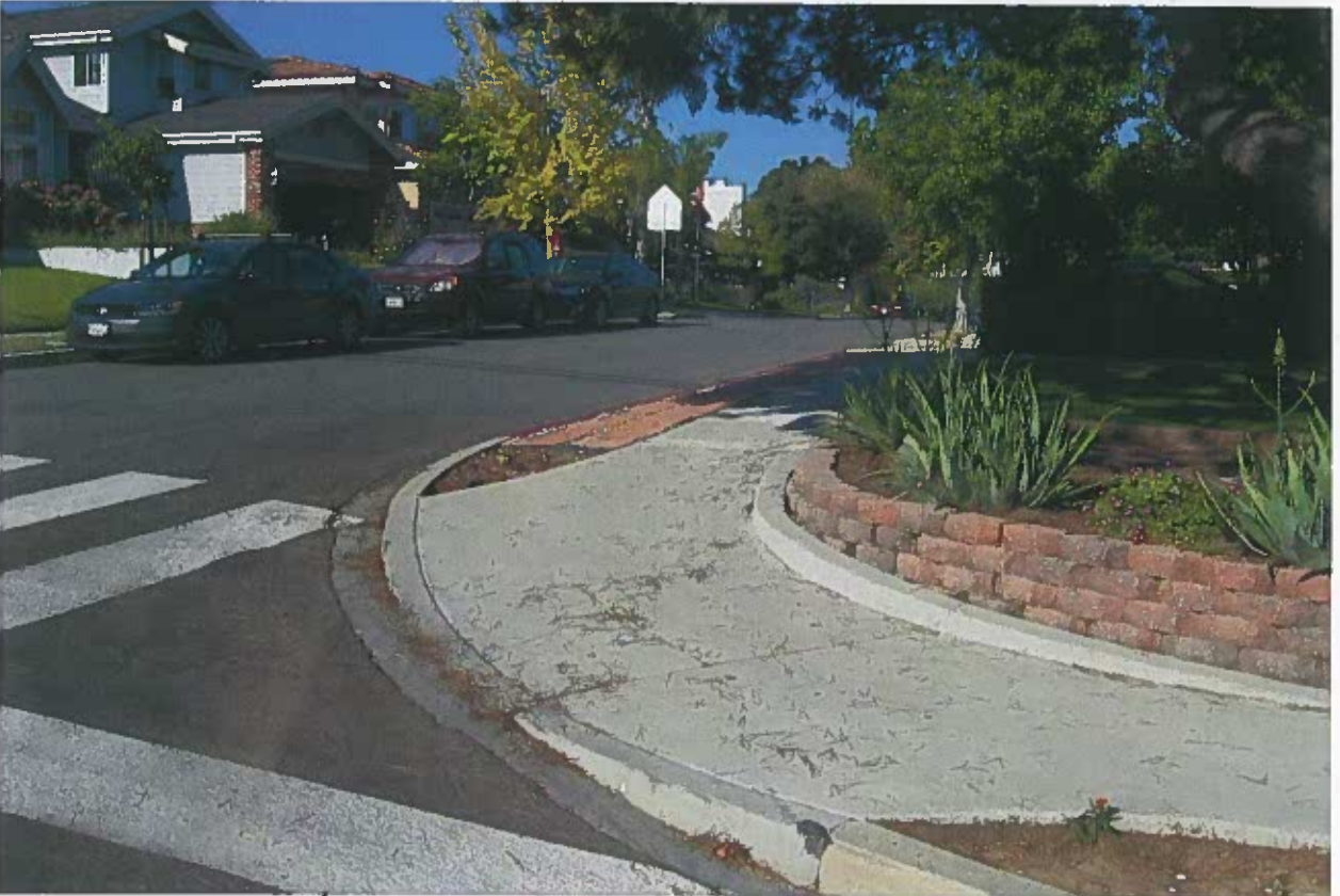
19 th Street (North Leg) at Rowell Avenue Looking West
