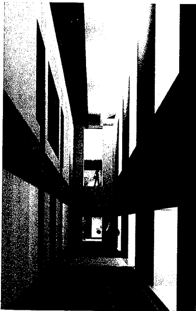
North Corridor View
