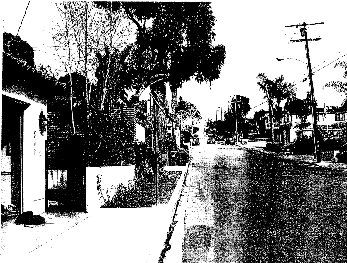
568 31 st Street – Recently Damaged and Removed
