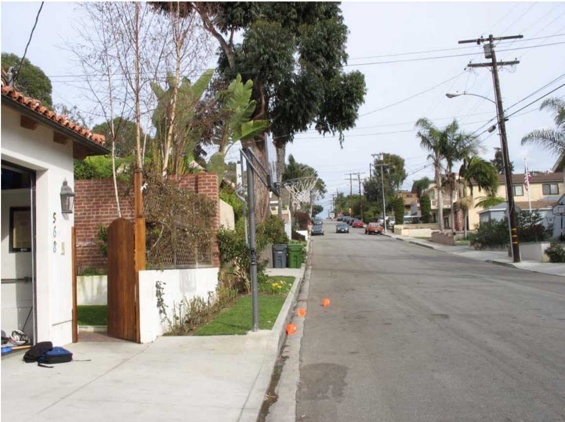
568 31 st Street – Recently Damaged and Removed
