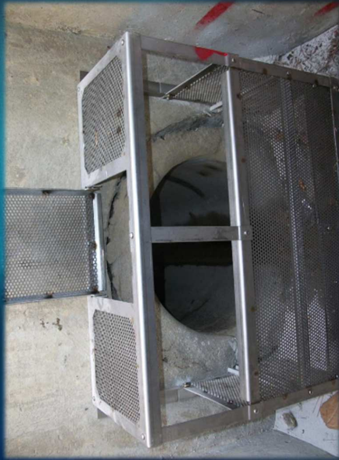
Connector Pipe Screens
