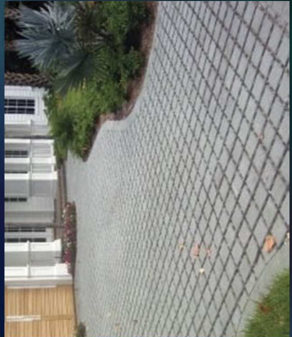
Permeable pavement application Photo Credit: Johnson Concrete
