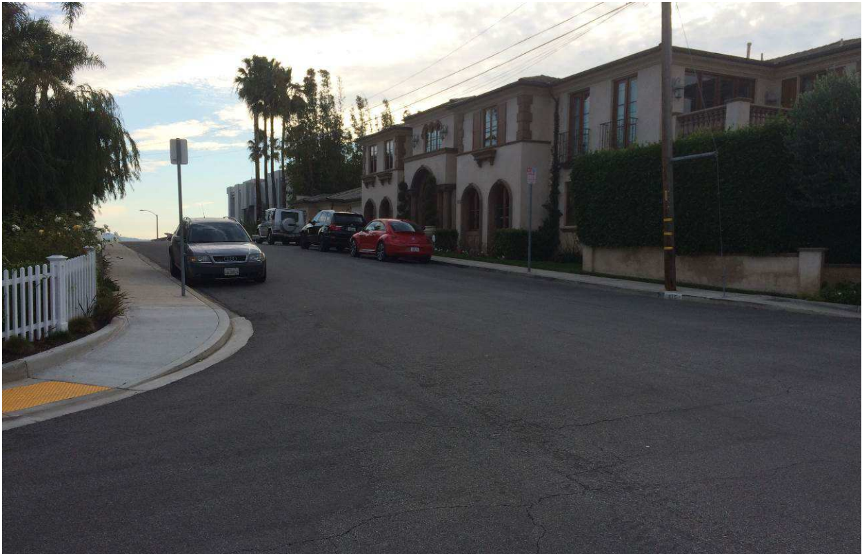
9th Street East of John Street Looking South
