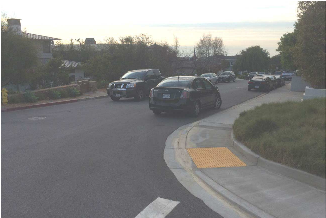
John Street North of 8 th Street at Looking West
