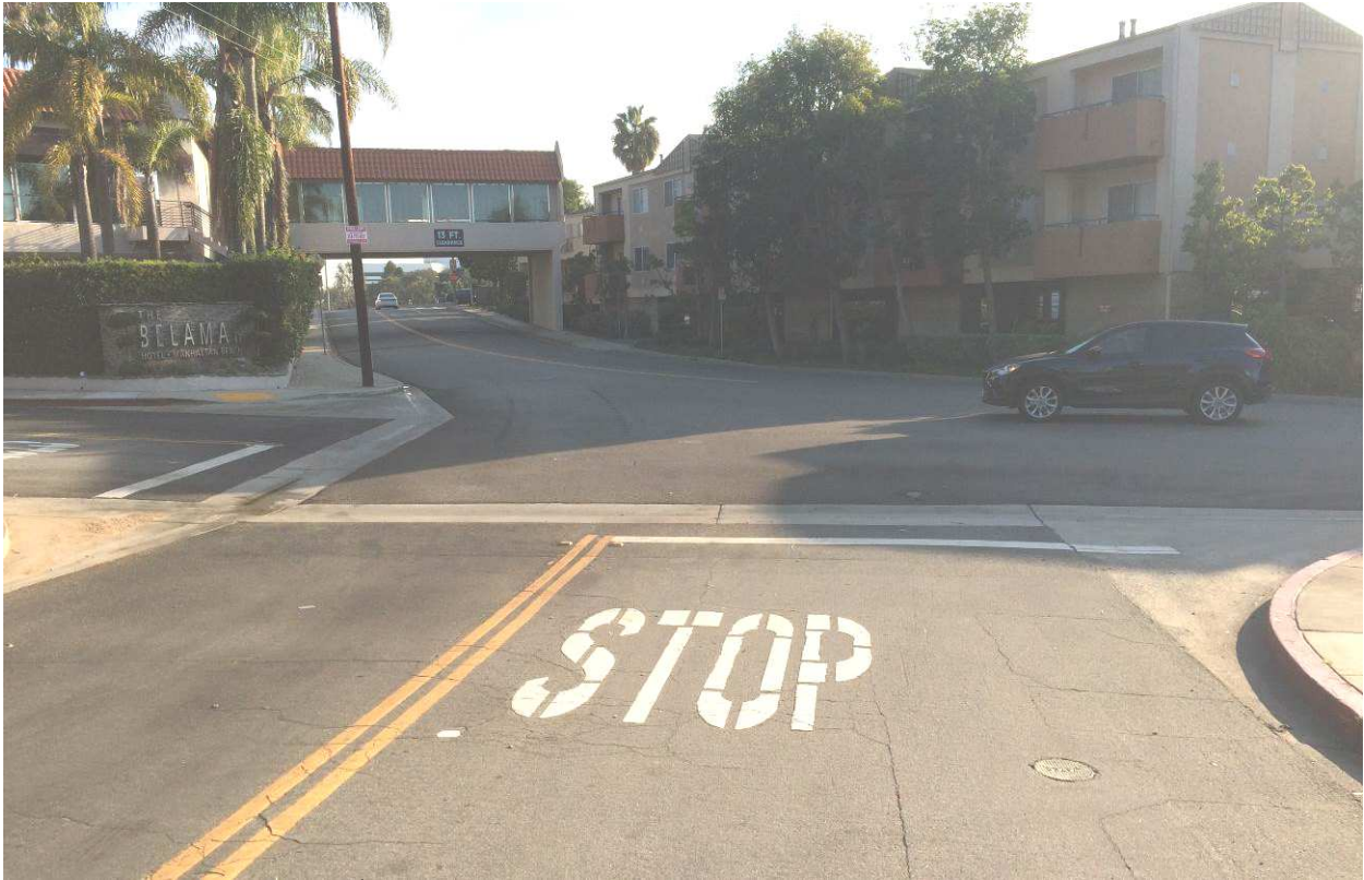
35 th Street West of Oak Avenue Street Looking East
