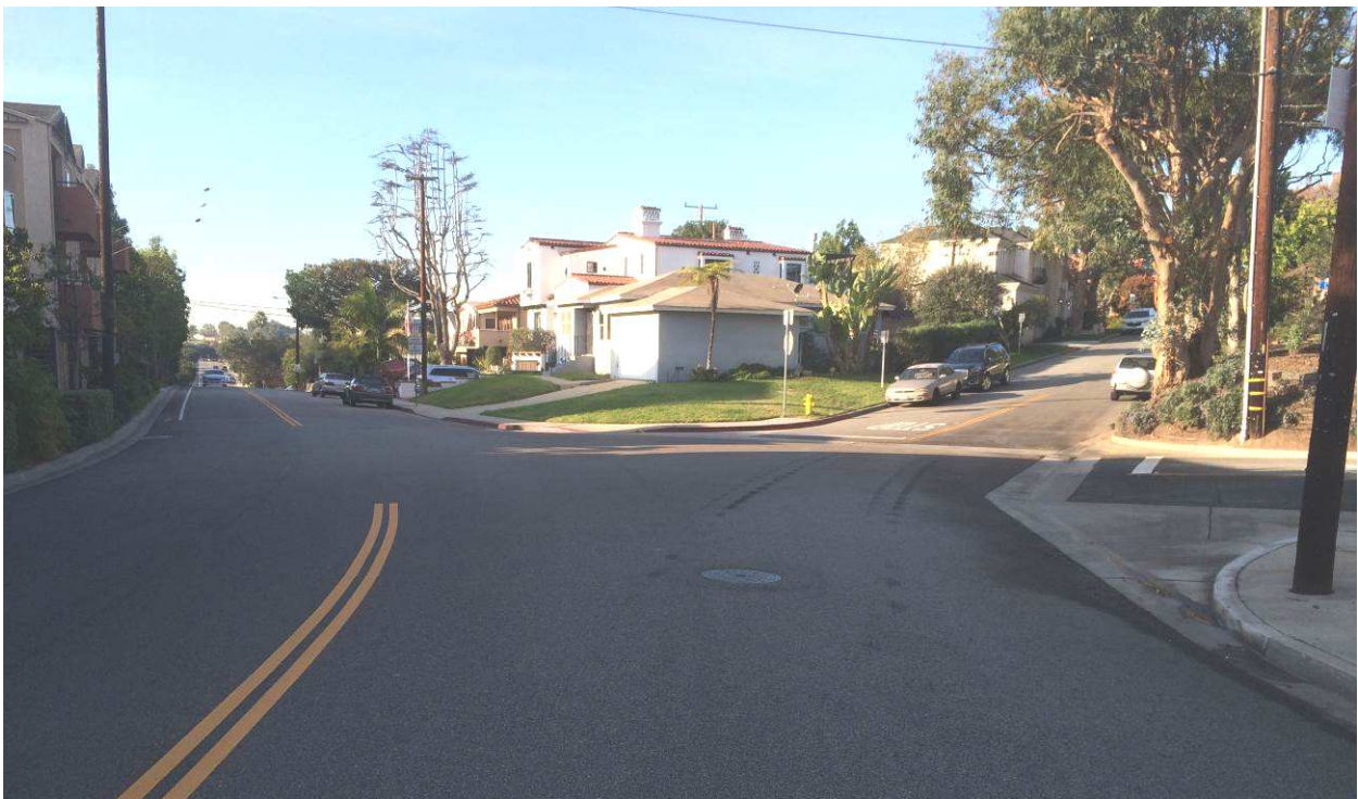
Valley Drive West of Oak Avenue Looking Southwest
