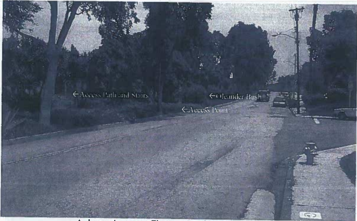
Ardmore Avenue at Flournoy Road Looking Eastbound
