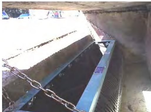
Figure 3-1. DrainPac™ catch basin insert.
