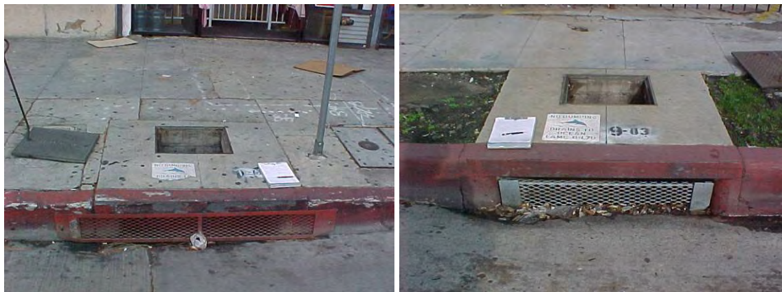
Figure 4-20. Curb inlet screens installed at two sites: FL003-F (left) and CC004-H (right).
