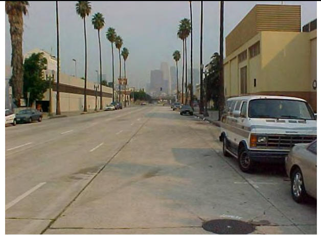
Looking upstream (~north) of CC-009F
