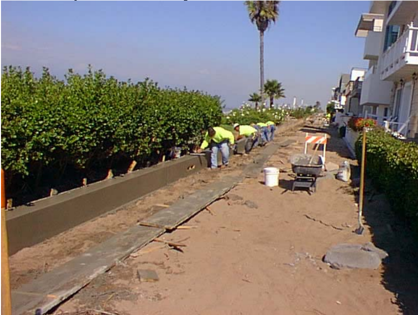
Construction of westerly concrete curb
