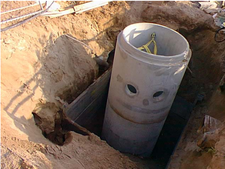
Installation of stormceptor unit at 32nd Street
