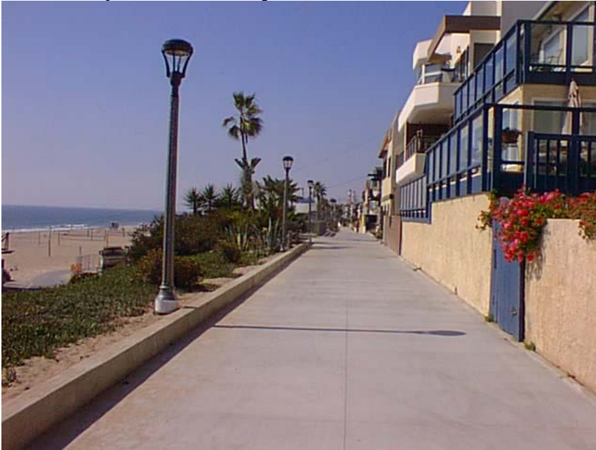
Completed Phase I Strand section
