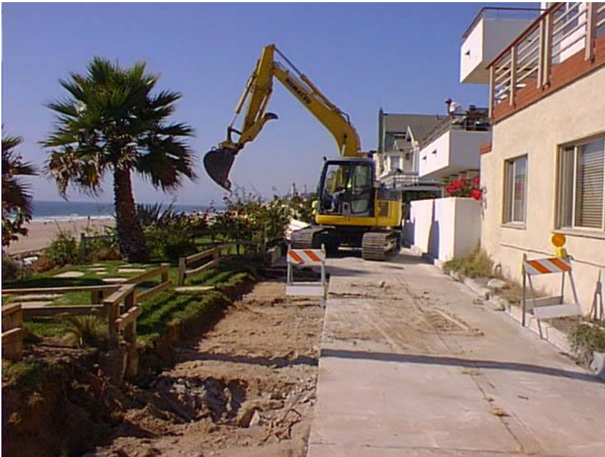
Existing curb and walkway demolition in tight quarters
