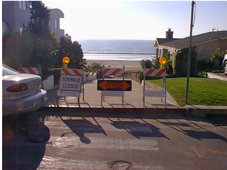
Typical pedestrian detour traffic control and signage
