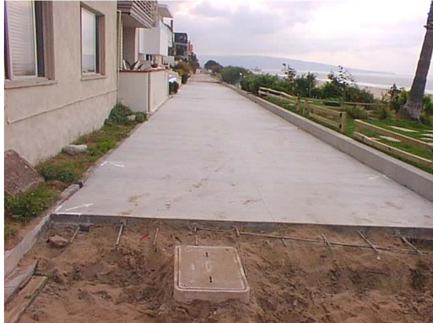
Completed Phase II concrete walkway section
