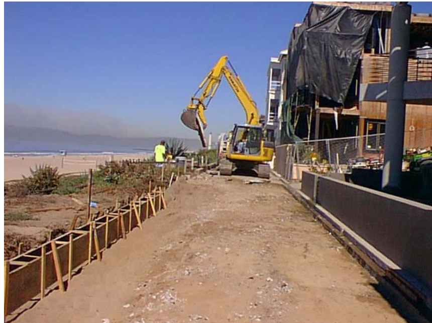
Existing concrete walkway demolition and removal
