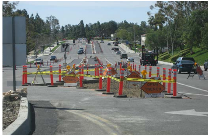
GOLDEN LANTERN ROADWAY WIDENING CITY OF LAGUNA NIGUEL
