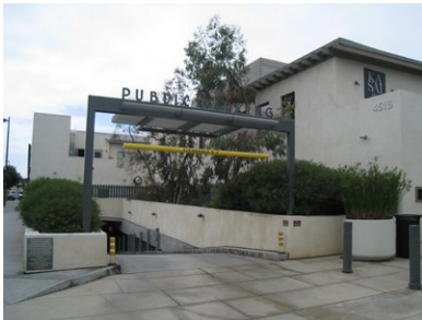
Figure 2.15 Metlox parking garage
