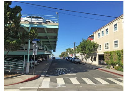
Figure 5.13 (top) Typical Tertiary Street Condition Figure 5.14 (bottom) Tertiary Street Type Cross Section
