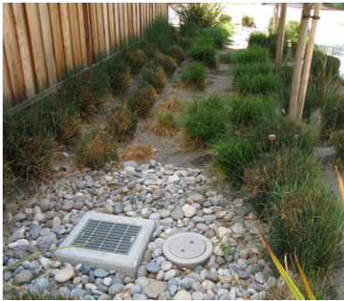
Figure 6.30 Vegetated bioswale filters stormwater
