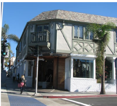
Figure 6.9 Corner entrance emphasized through unique articulation and materials
