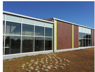
Figure 6.44 Green roofs absorb heat and rainwater
