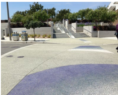
Figures 7.22 Concrete with recycled glass tends to last a long time with few maintenance problems
