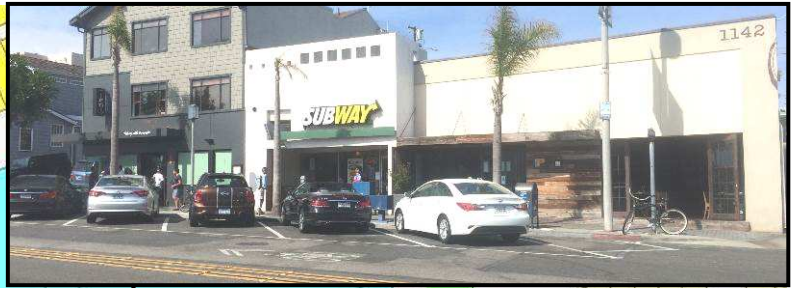
Existing (Location A)
