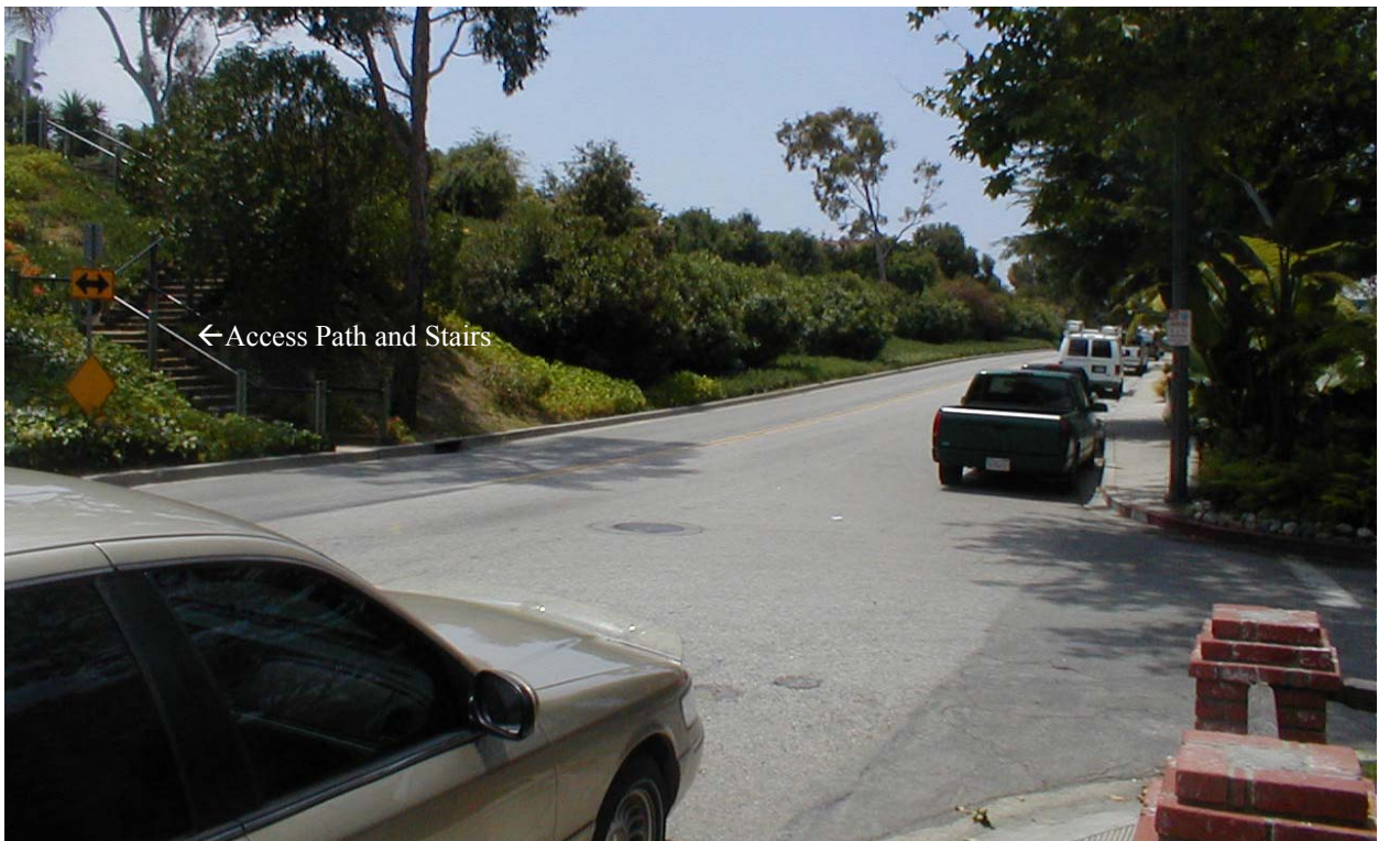
Valley Drive at Flournoy Road Looking West
