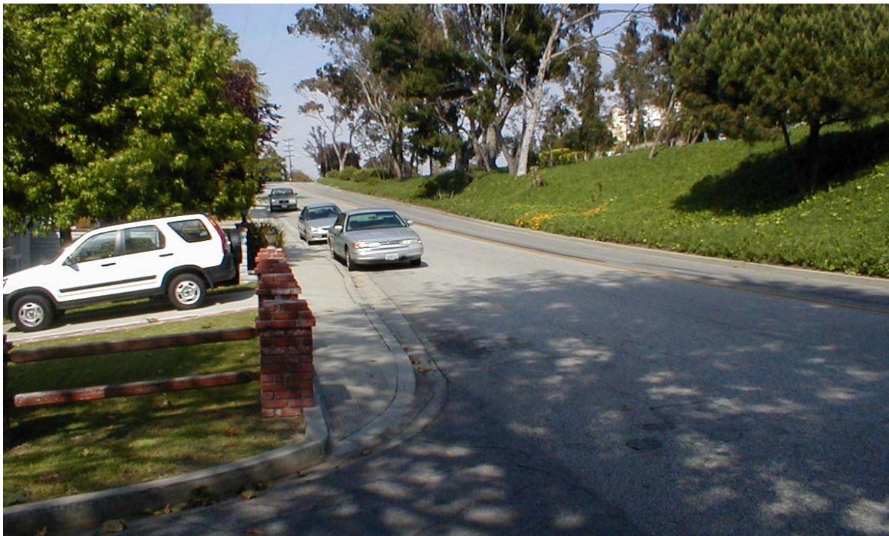
Valley Drive at Flournoy Avenue Looking East
