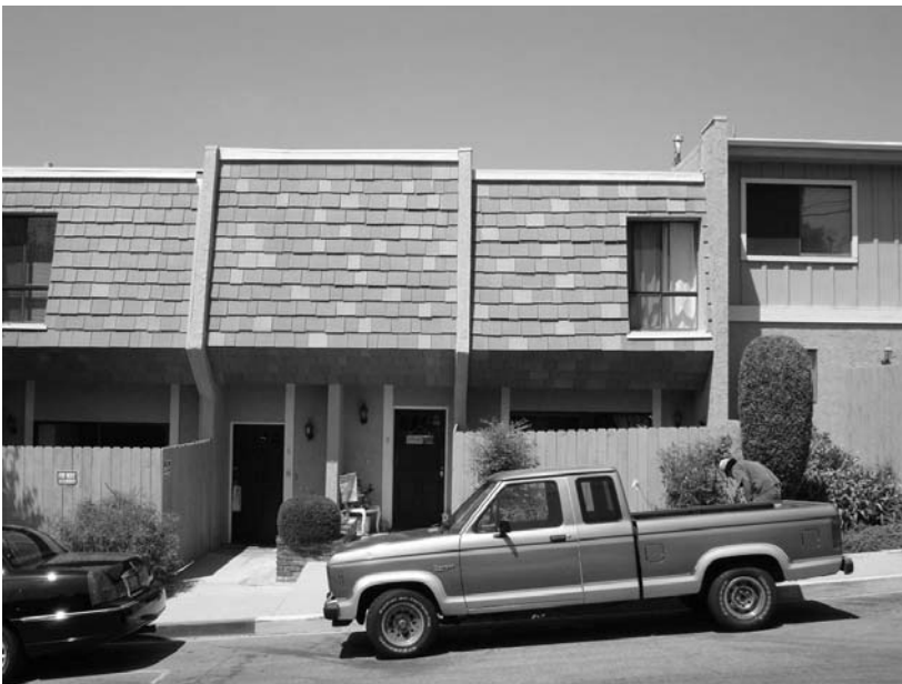
Front (North) view of our unit #5, unit #4 is on the right (East) side, 30" higher than unit #5. Satellite is not visible from the sidewalk on the other side of the street. Water will drain through downspout to street, like downspout on East side of unit #6 (left of #5).
