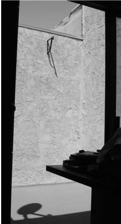
View of atrium from Master Bedroom facing NE corner. Unit 4 atrium is on other side of East (right-side) wall which is 30" higher than our roof.
