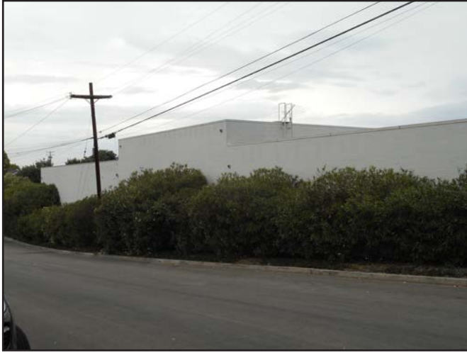
View 4: View of project site from Larsson Street, looking east.
