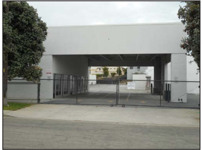
View 2: View of the project site from 8th Street.
