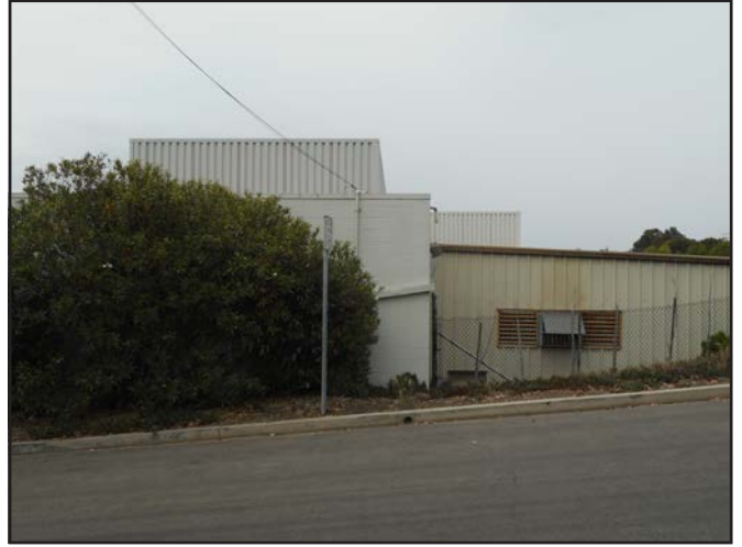
View 5: View of project site from Larsson Street, looking east.
