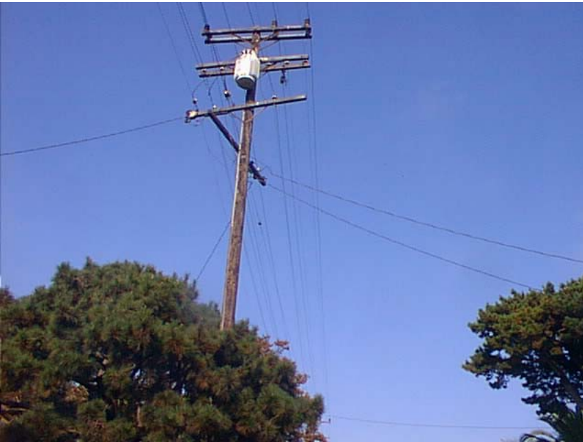
BELOW: Looking eastbound on 35 th Street
