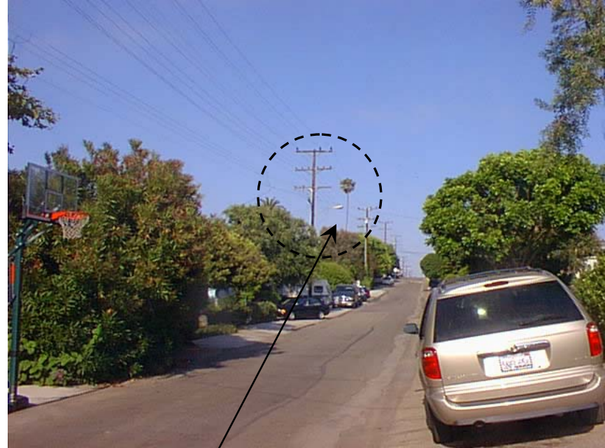
ABOVE: Existing Streetlight on 35 th Street
