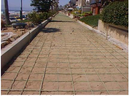
Installation of steel reinforcement for concrete walkway
