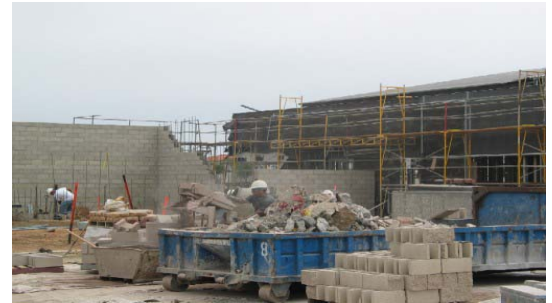
Below: Workers erect the masonry walls for Animal Control kennel.
