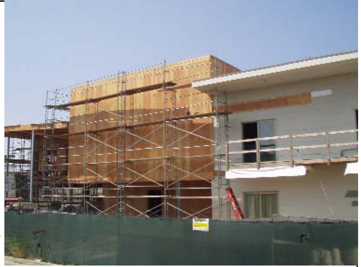
Above: Scaffolding around the exterior of Shade Hotel.
