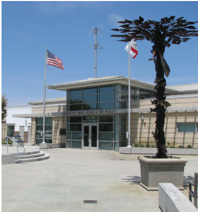
Figure 8.3 The Police & Fire Facility
