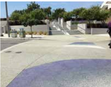
Figure 2-39 Concrete with recycled glass tends to last a long time with few maintenance problems
