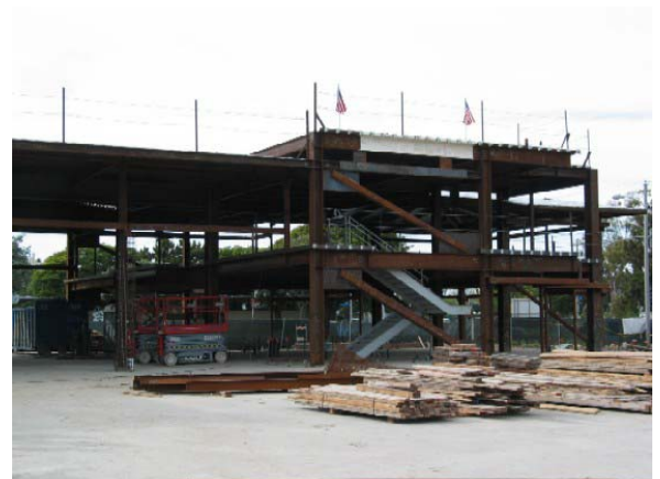
Above: Steel skeleton of the Fire garage
