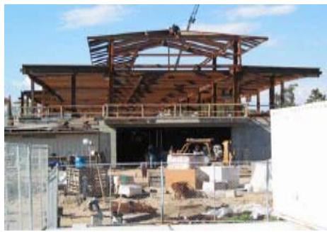
March 2005: The structural steel is put into place.
