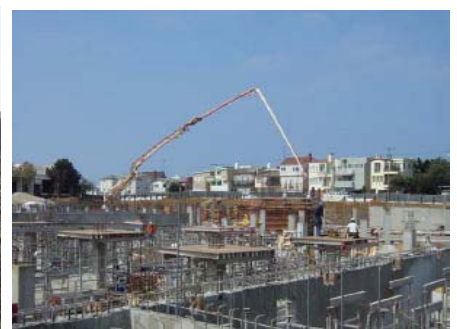
November 2004: Foundation walls and deck supports are in place.
