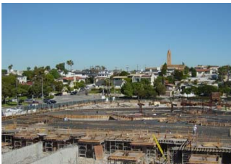
February 2005: The elevated deck being formed.
