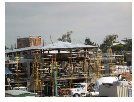
May 2005: The skeleton of the structure is in place.
