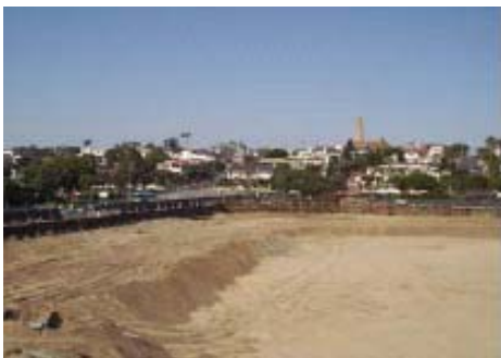
April 2004: The excavated footprint of the new safety facility.
