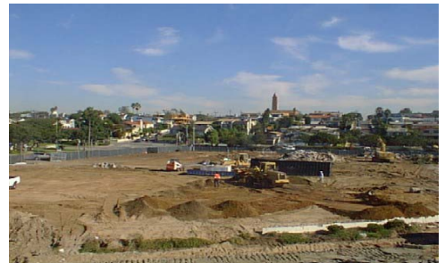
May 2004: Site Excavation takes place.
