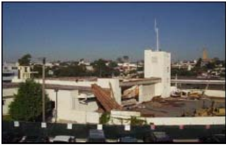
December 2003: Demolition of the old buildings.
