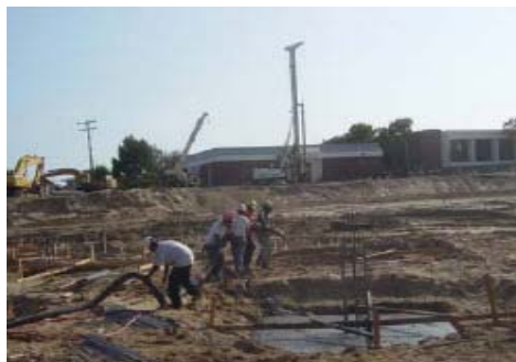
July 2004: Concrete foundation pours.
