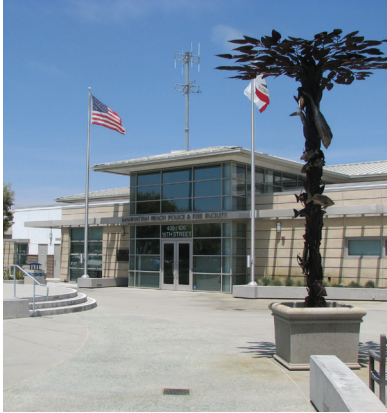
Figure 8.3 The Police & Fire Facility
