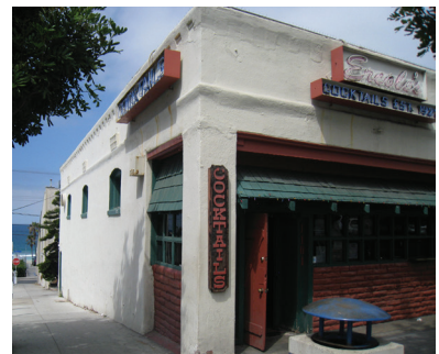
Figure 6.25 1101 Manhattan Ave is the oldest commercial building in the Downtown
