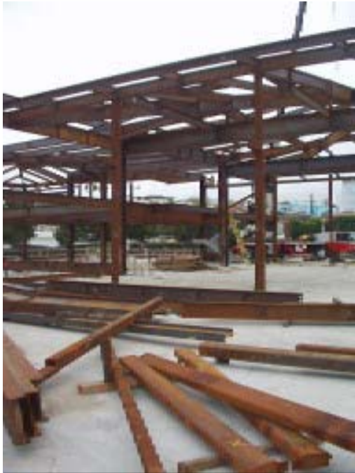
Above: Steel beams for the skeleton of the Police & Fire Facility.
