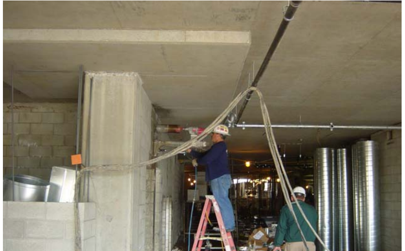
Above: Workers installing sprinkler piping in the Police & Fire Facility
