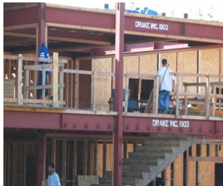
Far Right: Structural Steel being erected for the Police & Fire Facility
