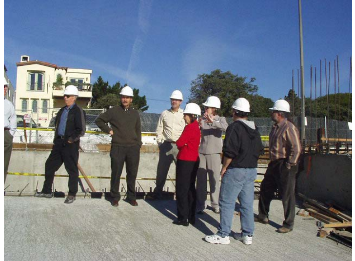
Above: The Construction Issues Committee touring the Police & Fire Facility Site
