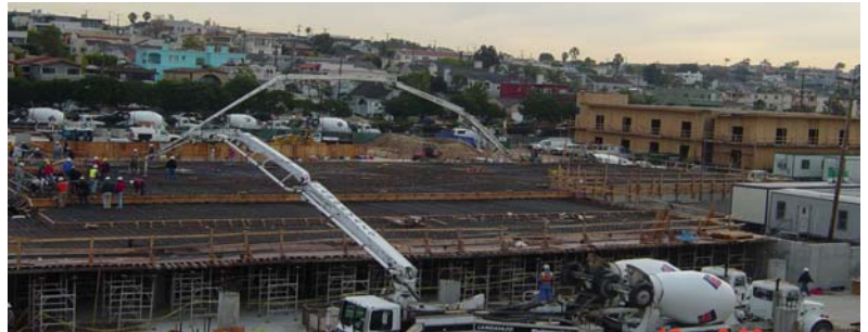
Top Page: Masonry work at the Police & Fire Facility
