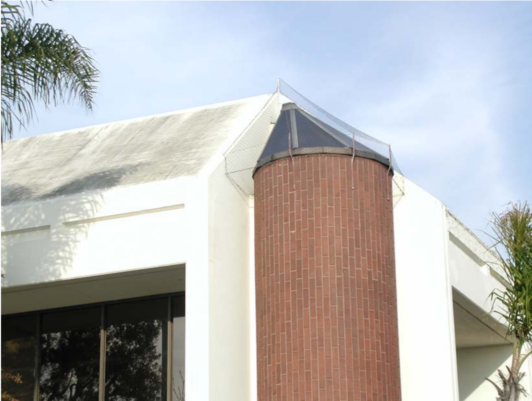
Existing southwest corner
