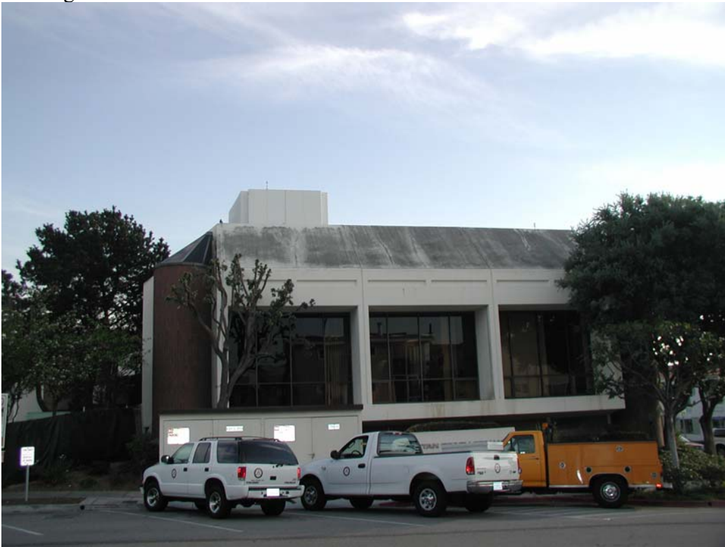
Existing northeast corner
