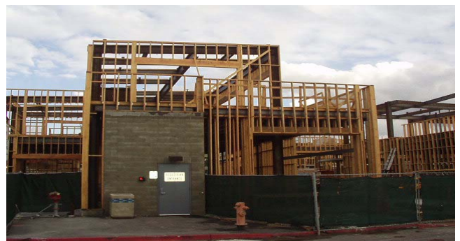
Below Right: The wood framing of buildings along Morningside above a parking garage pedestrian exit.
