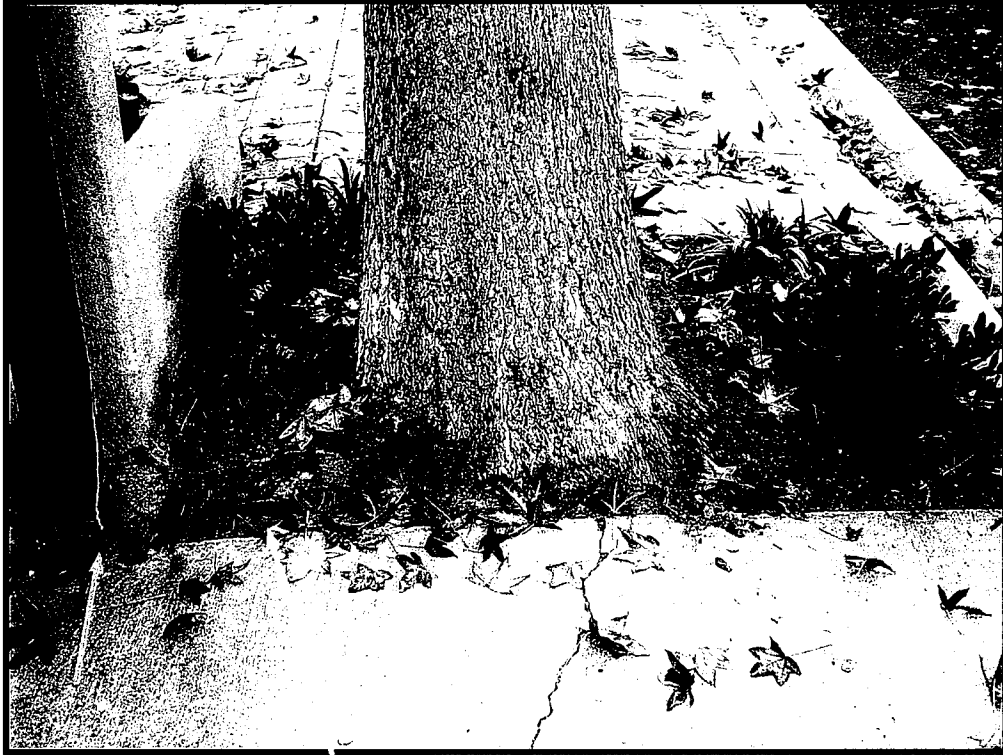
Figure 1.3 (above), note the damaged root and the crack in the driveway apron; it is likely that roots were cut prior to installing the wall footing; Figure 1.4 (below), note the damage to the street surface; any large roots cut on this side will likely reduce structural stability since this tree is already leaning.
