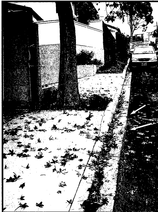
Figure 1.3 (above), note the damaged root and the crack in the driveway apron; it is likely that roots were cut prior to installing the wall footing; Figure 1.4 (below), note the damage to the street surface; any large roots cut on this side will likely reduce structural stability since this tree is already leaning.
