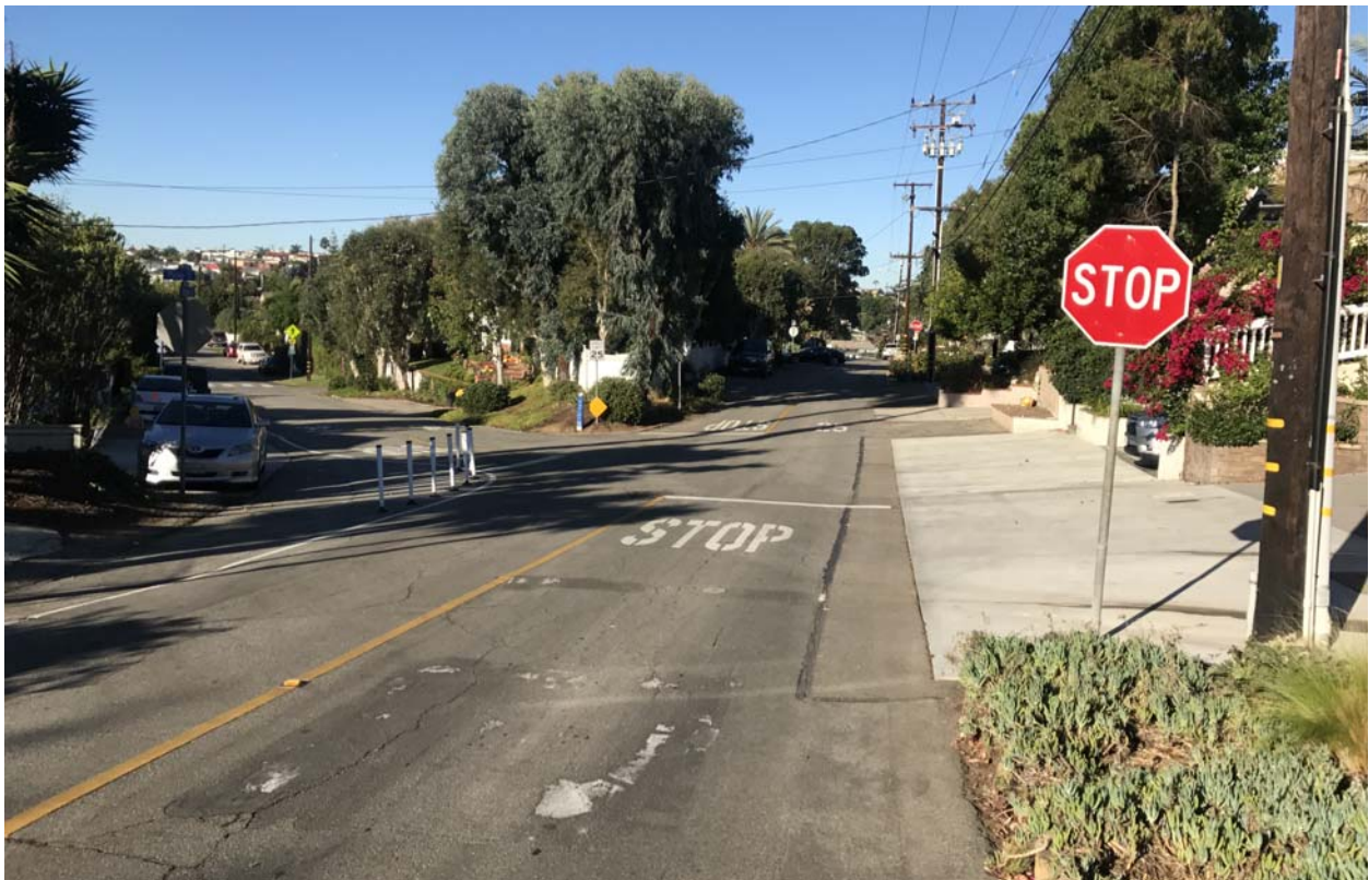
Marine Avenue at 25 th Street Looking West (Intersection Realignment)
