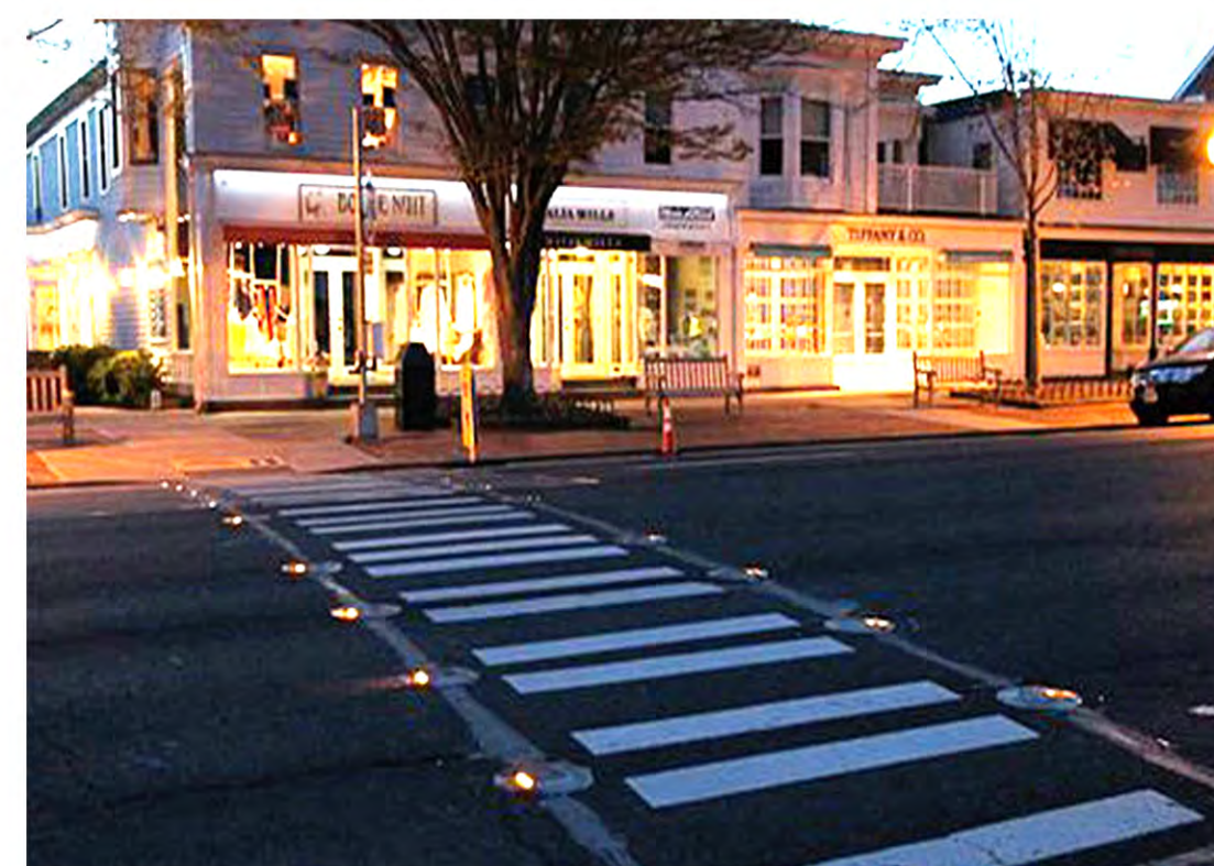
In-Roadway Warning Lights
