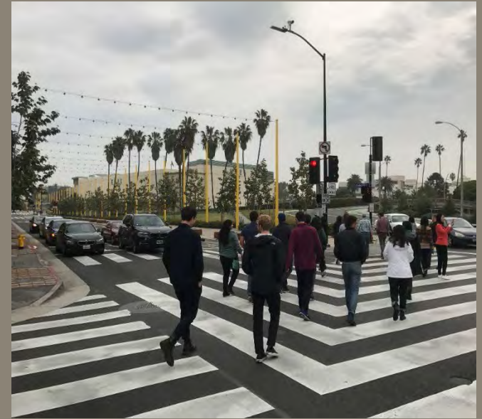
All-Direction Pedestrian Scramble Crossing Treatment, Santa Monica
