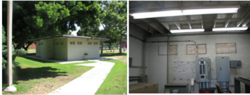
Old Restroom turned into Offices and Storage
