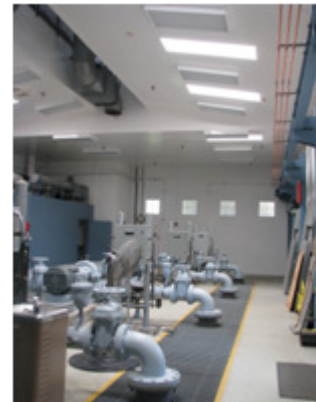
Pumping Station Daylighting
