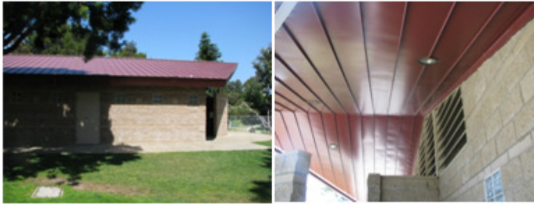
New Restroom Facility
