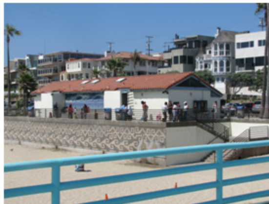
Beach and Restroom Facility
