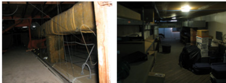
Attic Space in Joslyn C.C.
