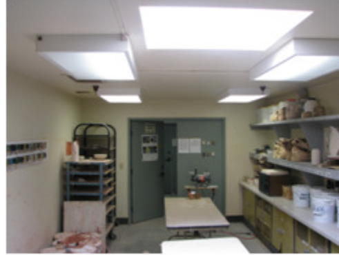
Ceramics Room with Skylight
