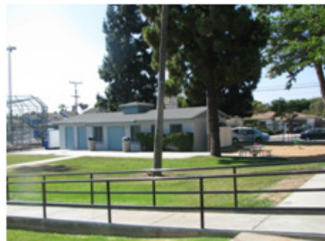
Restroom /Playground Bldg
