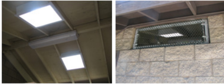
Beach Restroom Daylighting
