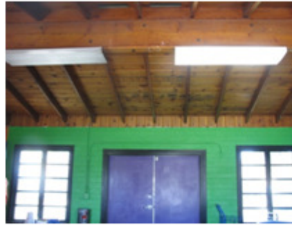
Restroom Bldg/Playground Room
