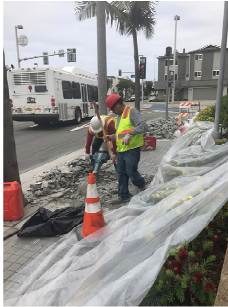
Preparation Work— Removal of gray tiles
