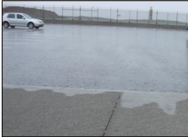
Permeable Pavement Application Los Angeles World Airports Parking
