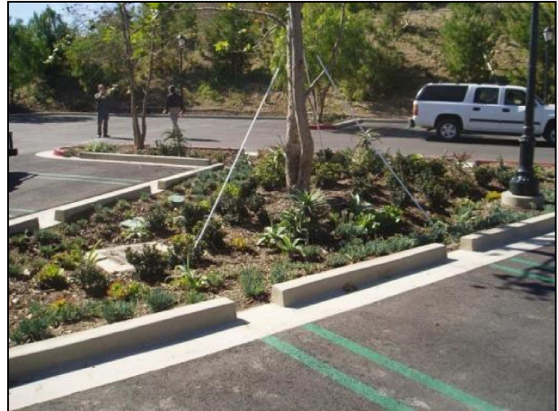
Bioretention in a Parking Lot
