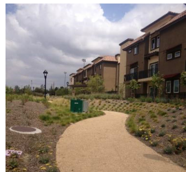
Underground Cistern Taylor Yard
