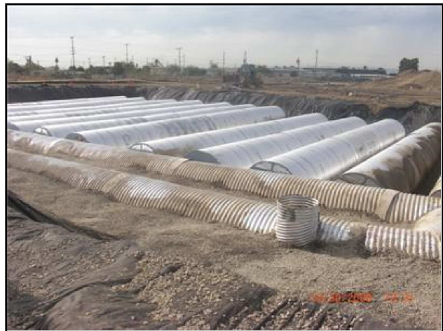
Underground Infiltration Units Lowe’s, Pacoima
