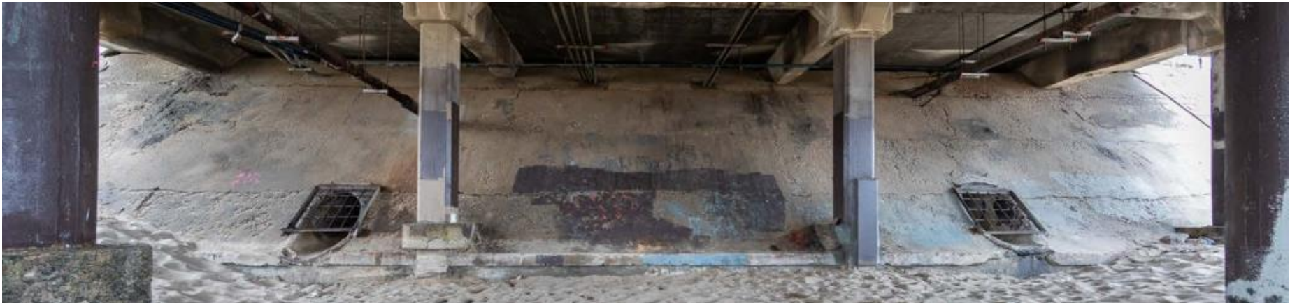
Stormwater outfalls
