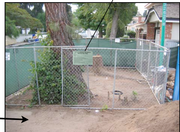
Fenced Area Large As Possible to Protect the Root Zone
