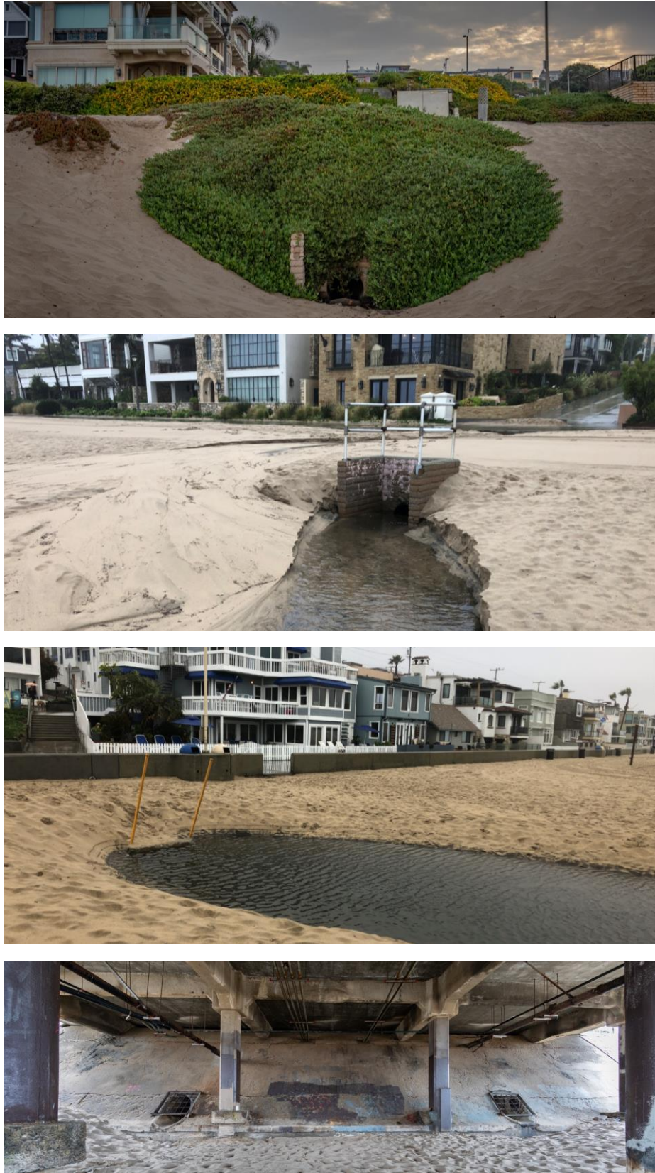
Figure 3-8: Stormwater Outfalls onto the Beach that Drain Higher Areas of the City
