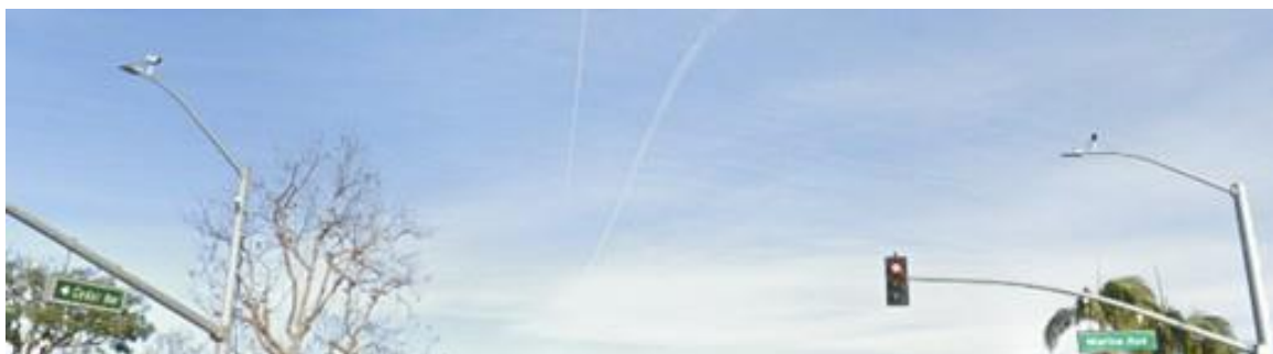
Existing Video Detection Might be Upgraded for Pedestrians and Bicyclists
