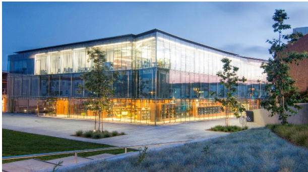
Photo: Sentech Architectural Systems
